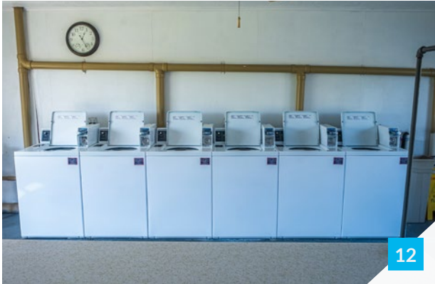
LAUNDRY FACILITY INTERIOR
