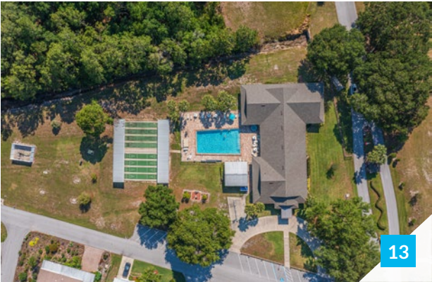
AMENITY CENTER AERIAL
